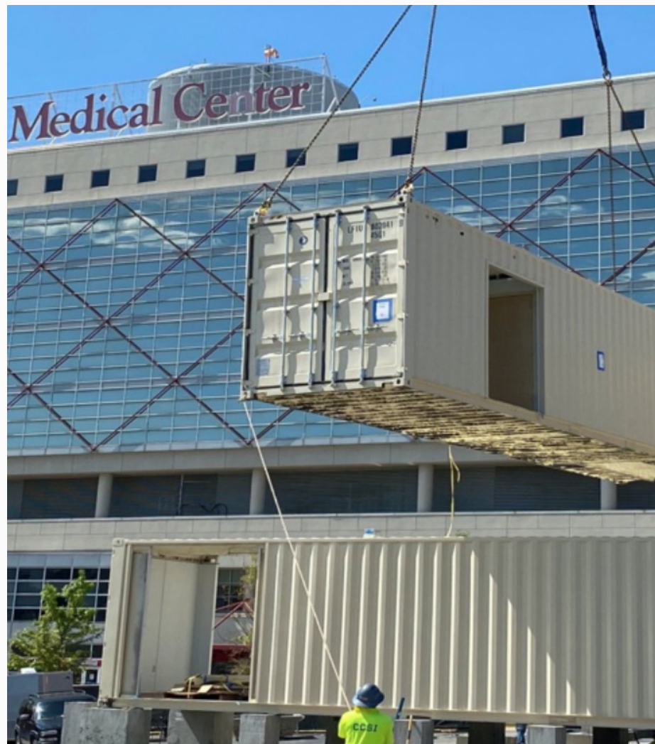
Figure A3-1: Modules During Site Installation
