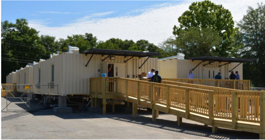
Figure A3-2: Temporary Modular Hospital Designed for GEMHSA
